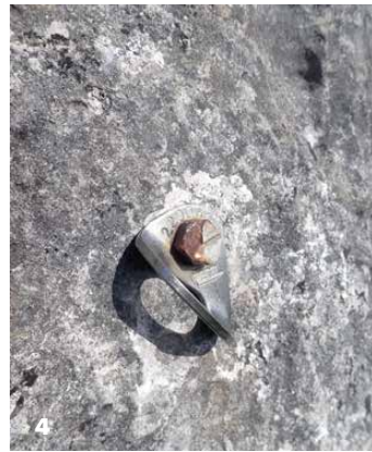
1. Hole-drilling and cleaning equipment carried on abseil. 2. Glueing equipment carried on abseil. 3. It's a dirty job but someone has to do it if we're going to sport climb. 4. A good hanger with a non-compatible bolt resulting in mixed metal corrosion. Who knows what's underneath. 5. 1980's tat with lichen camouflage. 6. Checking the hang of a quick draw before beginning the glueing process.
